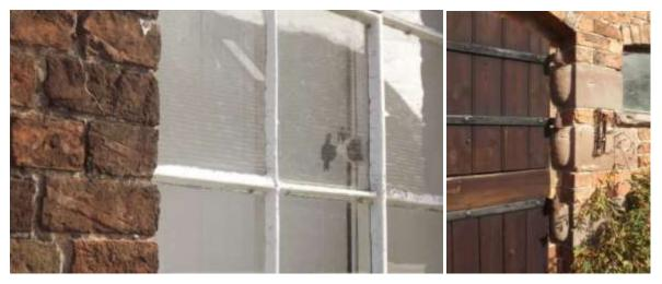
Figure 9 Cast iron 'hand' window catches and moulded stone door hinge holders
