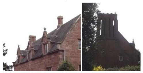
Figure 8 Roof dormers and finials at Forton House and chimney stacks to Forton Hall
