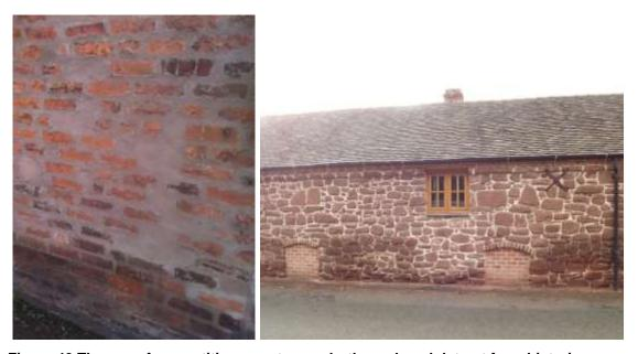
Figure 40 The use of cementitious mortar can both mask and detract from historic masonry
